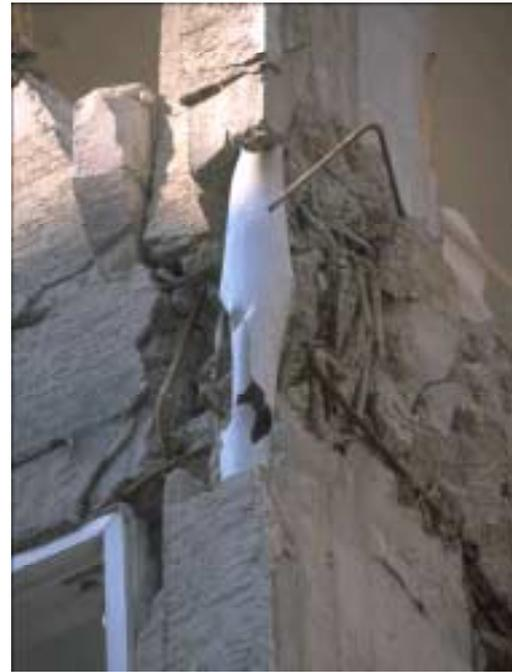
Figure 5. Disintegration of a poorly detailed beam-column joint
