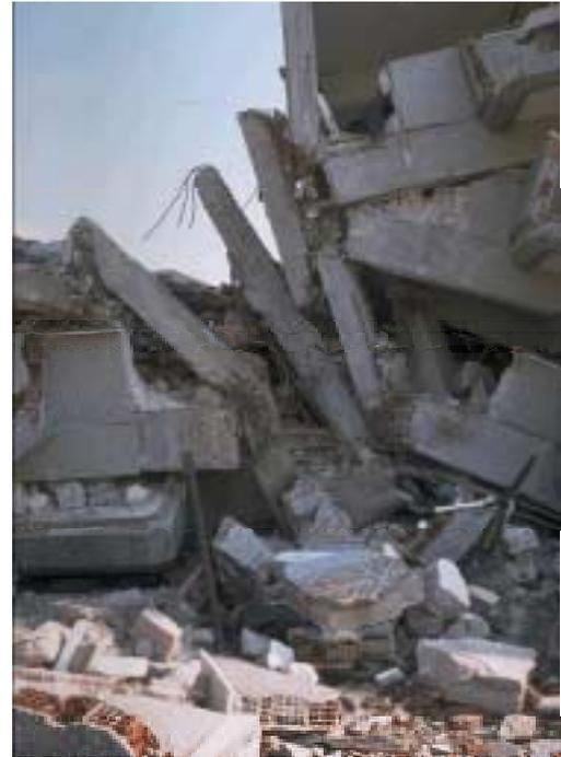
Figure 2. Total disintegration of a RC frame (Kocaeli earthquake, 1999)
