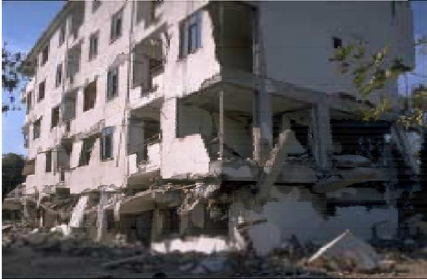
Figure 3. Soft story mechanism formed after the fall out of the infills in the lower two stories (the situation never considered in the design)
