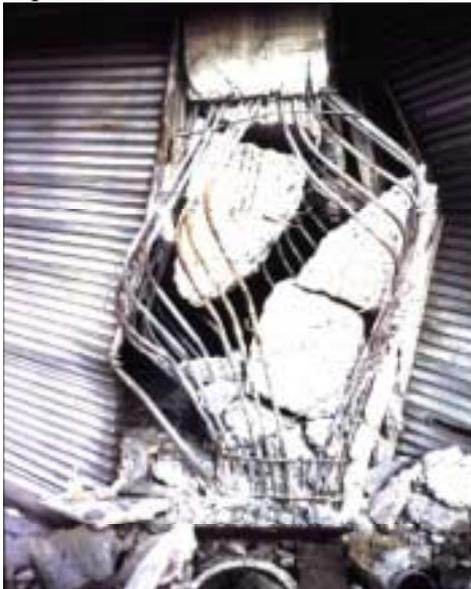
Figure 4. Combined shear – axial compression failure due to the lack of confinement
